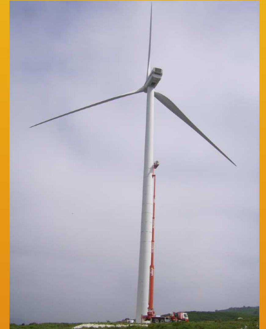
WIND TURBINES MAINTENANCE AND REPAIR
