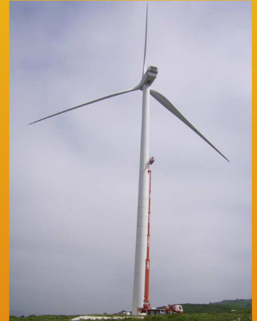
WIND TURBINES MAINTENANCE AND REPAIR
